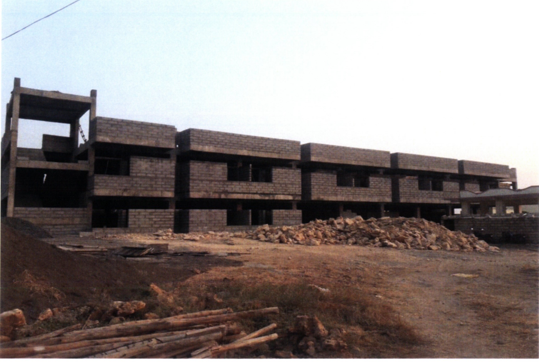
LADIES HOSTEL—UNDER CONSTRUCTION
