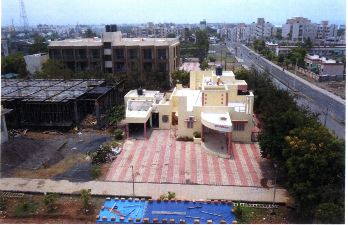
VICE-CHANCELLOR'S BUNGLOW & GUEST HOUSE UNDER CONSTRUCTION
