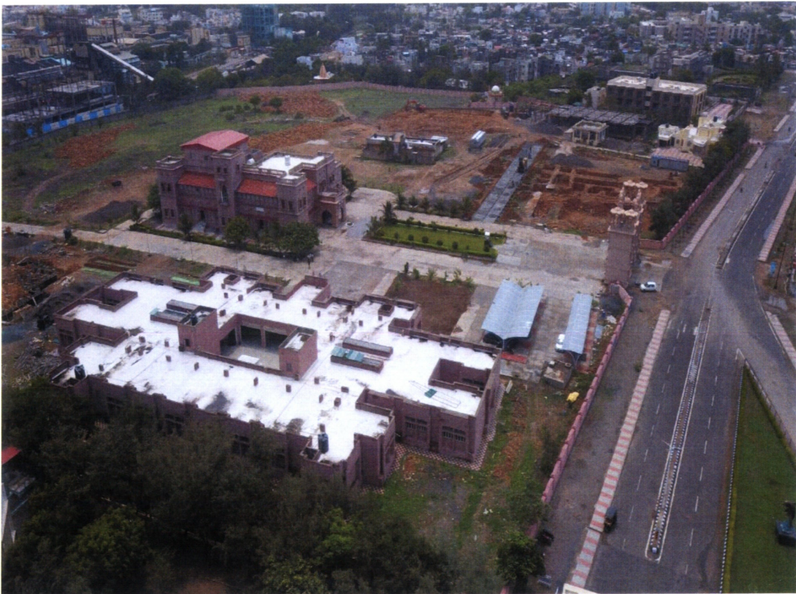
BIRD'S VIEW OF THE CAMPUS
